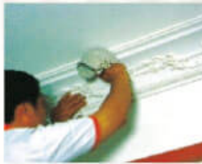
9. Cleaning overflowed glue with the waterish cloth;
