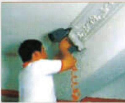
5. Using pressure gun for nailing, if the wall is too strong then use the steel nail;
