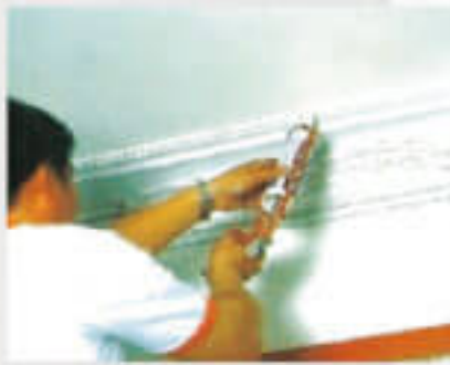
8. Apply the filler (Silicone or Plaster) to fill up the gaps;
