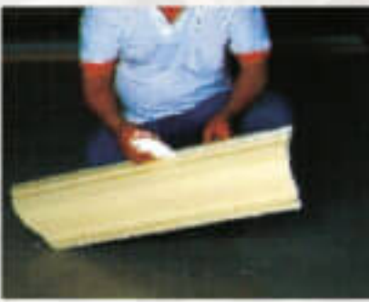
4. Apply silicone or adhesive on both backedge of the cornice, which will be contact with the wall and ceiling;
