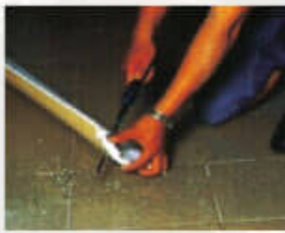
3. Saw at the marked point of the cornice, and better to cut more 5mm than the marked point;
