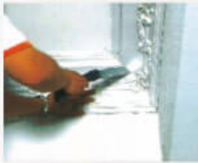
6. The joints between the cornices can be amended with the saw or the sandpaper;
