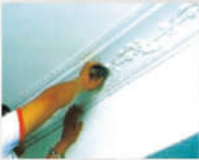
10. Allow to dry, sand smooth with sandpaper and finished with paint.
