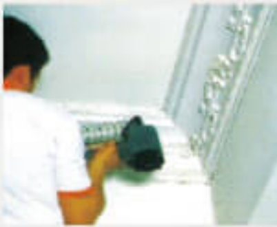
7. Fasten the cornice with the pressure gun or steel nail, and fill the nail holes with plaster;
