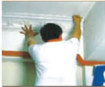
1. Establish a horizontal reference line on wall for the cornice;
