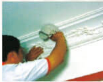
9. Cleaning overflowed glue with the waterish cloth;
